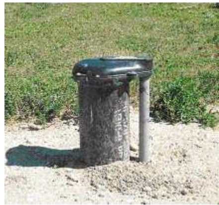
A properly cased and sealed well protects water quality.
